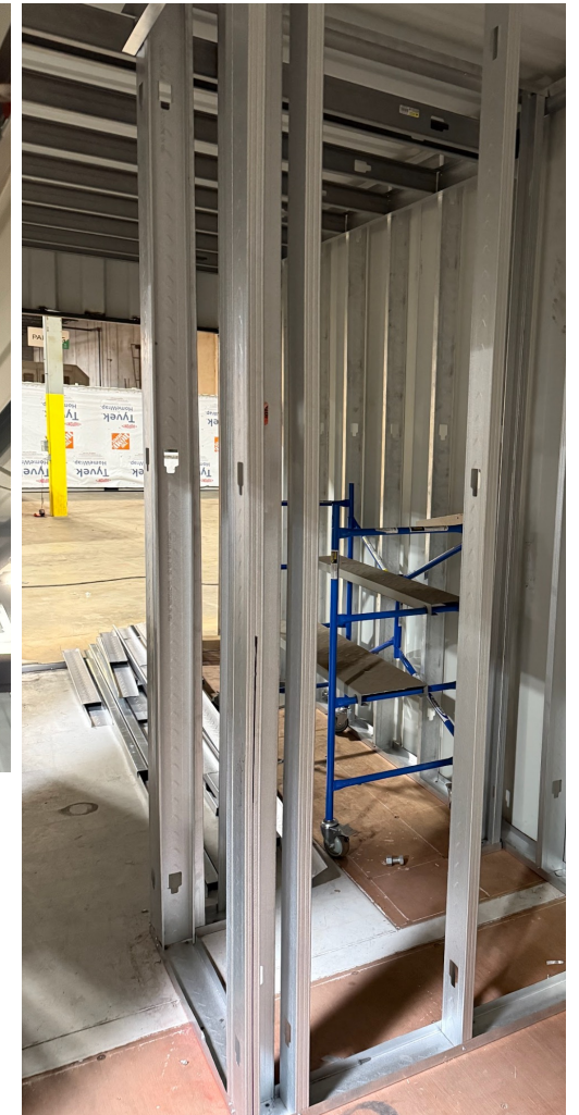
Metal Studs to Eliminate Mold
